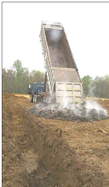
Figure 1. Excavated trench and a load of municipal biosolids
