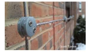
Care should be taken in both the planning and installation of a green façade cable system, as proper anchoring and cable spacing are vital to sustained welfare of the trellis.
