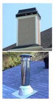
Two examples of prefabricated chimneys.
