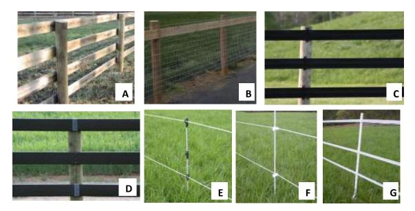
**Figure 2**. Perimeter and internal fencing types used at the site A) Four rail wood board fence with pressure treated pine boards, B) 2 x 4" woven wire mesh with pressure treated pine top rail, C) Four HorseRail® polyethylene with high tensile wire, and D) Four rail Palladium with plastic covered treated lumber, E) Two rail 1/4" electric braid with fiberglass step-in post, F) Two rail 1/3" electric braid with drilled plastic post, and G) Three rail 2" electric tape with plastic push in post.
