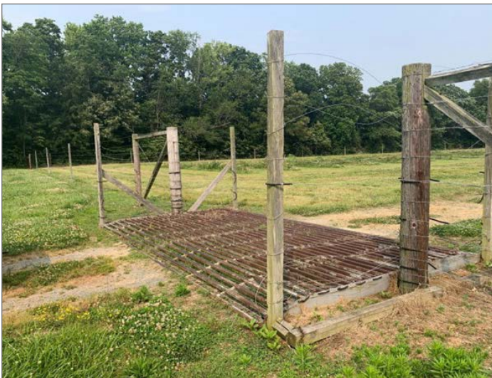
Figure 25: A cattle-guard style gate structure that allows easy entry and exit of farm machinery while excluding deer. Note the T-shaped ends that prevent deer from jumping at a diagonal approach. In this case, electrified strands are also placed between the cattle guard bars along the first half of the entrance. Photo by Chris Cochran.
