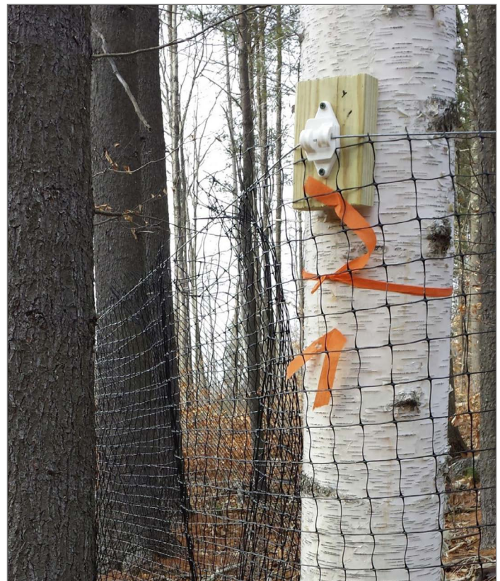
Figure 20: Plastic mesh fencing using existing trees as fence posts and wooden battens to prevent wire from growing into trees. Photo Credit: Smallidge et al. 2017, Cornell Cooperative Extension
