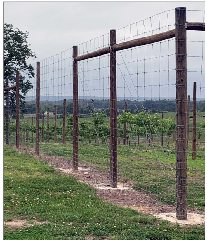
Figure 21: 8' permanent wire fence can effectively prevent deer entry. Photo by Luke Macaulay.
