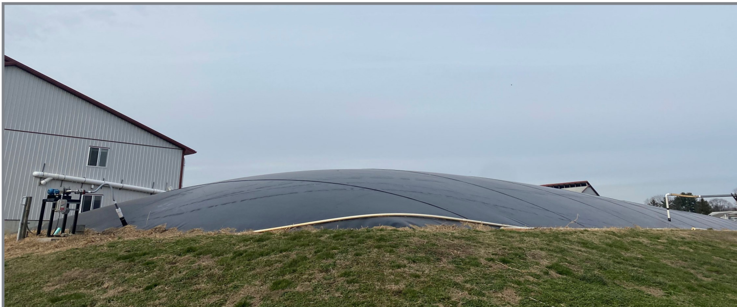
Covered lagoon anaerobic digester at Kilby Farm in Cecil County, MD. Photo: Amro Hassanein
