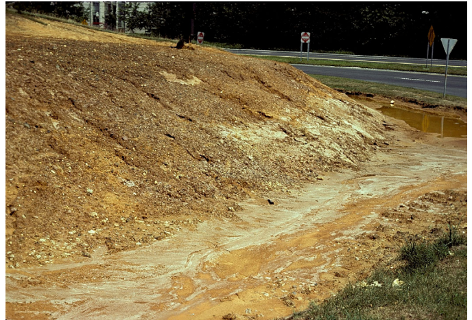
Construction site for ornamental flower meadow
