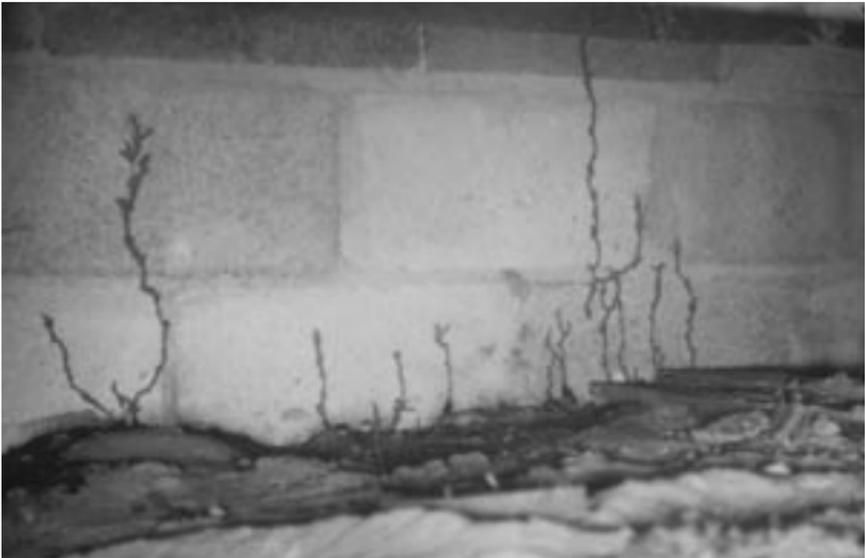
**Figure 4.** Termite tubes on the foundation of a structure.
