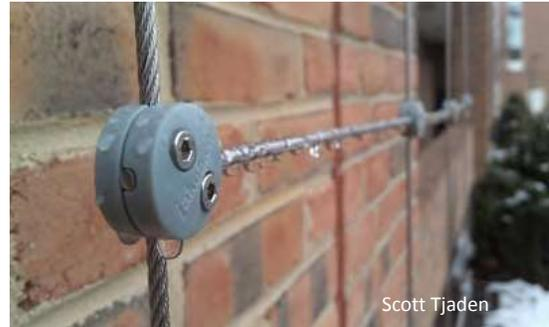
Care should be taken in both the planning and installation of a green façade cable system, as proper anchoring and cable spacing are vital to sustained welfare of the trellis.
