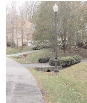
**Grass swales** are an alternative to the curb and gutter system. Grasses or other low-growing vegetation are planted to reduce runoff velocity and allow filtration, while high-volume flows are safely channeled into a storm sewer or retention basin. Native plant species such as white ash, red cedar, chokeberry, sunflowers and switch
