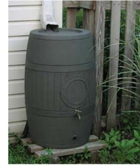
Stormwater can be collected from rooftops by diverting downspouts into rain barrels. Rain barrels help slow the flow of runoff from impervious surfaces and store water for future landscape uses. Multiple rain barrels can be linked together to increase storage capacity.
