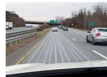
Anti-icing or pre-wetting with salt brine prior to storms is one of several salt management practices used to reduce salt application.
