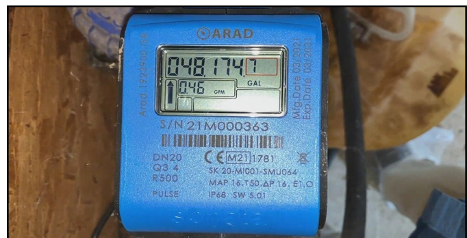
Figure 4. Tunnel fan end water meter
