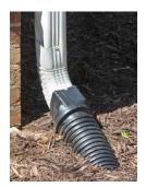
You can connect flexible tubing to your put the tubing underground or on the soil surface to into garden areas rather than on impermeable as driveways, sidewalks, and streets. (photos author)
