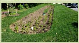
Micro-Bioretention: A Micro-Bioretention is a stormwater management practice that also serves as a landscape feature. It is composed of three layers: sand, soil, and an organic layer. Water filters through the system and is transferred through a perforated storm drain to the reforestation area. After a large rain event, this facility will drain within 2 days. A Rain Garden is similar except it does not have an underdrain.
