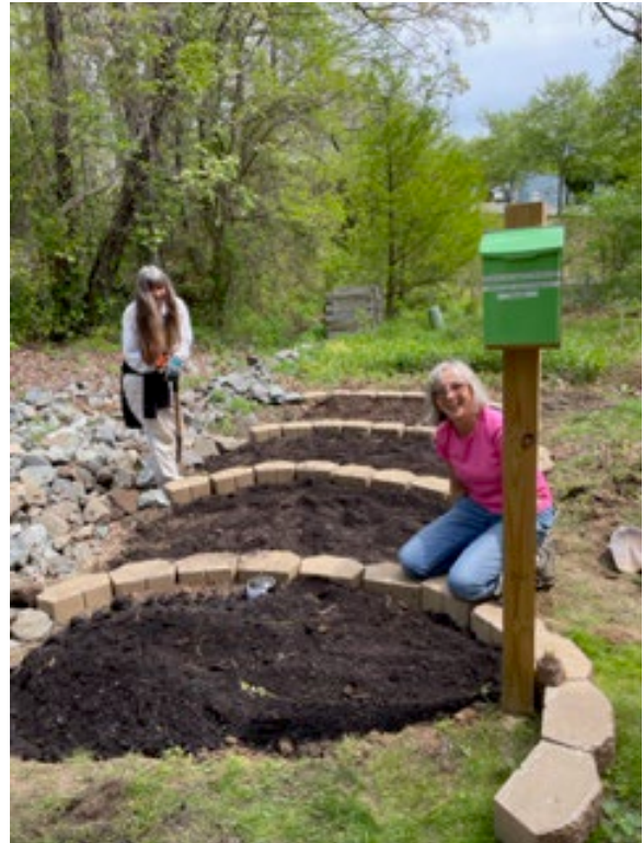
Calvert County Bay-Wise Master Gardeners constructing tiers to control stormwater runoff at their Extension office in Prince Frederick.
