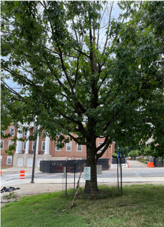
Fence circling the trunk of a tree in a construction area.
