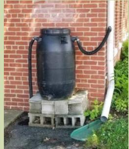
**Rain Barrels:** Rain barrels collect water from roof downspouts and store it for later use in the demonstration garden on site. Benefits of a Rain barrel: Can reduce water usage from municipal or well sources for gardening needs.
