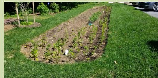
**Micro-Bioretentation:** A Micro-Bioretentation is a stormwater management practice that also serves as a landscape feature. It is composed of three layers: sand, soil, and an organic layer. Water filters through the system and is transferred through a perforated storm drain to the reforestation area. After a large rain event, this facility will drain within 2 days. A Rain Garden is similar except it does not have an underdrain.
