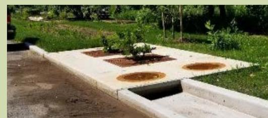
**Filterra:** In a Filterra, stormwater enters into the system from a curb opening and then is filtered through mulch and organic layers before being transferred out through a pipe system. These systems have high pollutant removal rates with a reduced footprint, are aesthetic appealing and are easy to maintain.
